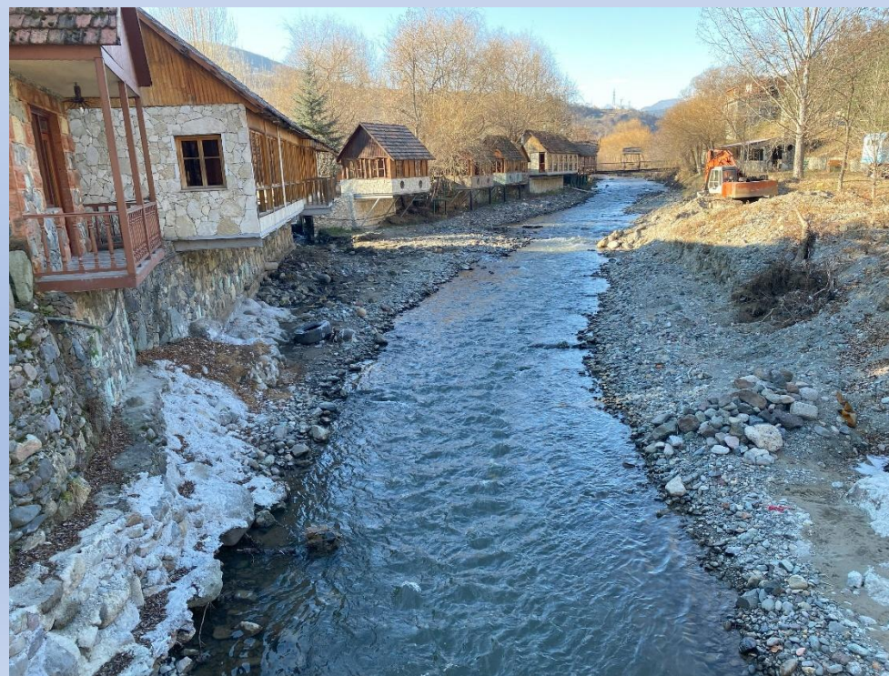
Construction at the river bed
